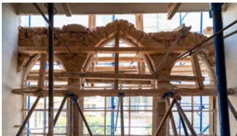
The dismantled arches, and their re-installation, D. Mrad
