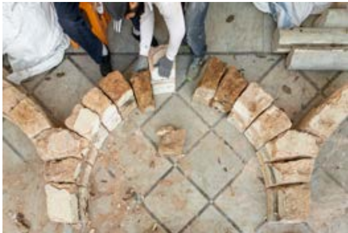
Laying of the fallen sandstones, D. Mrad
