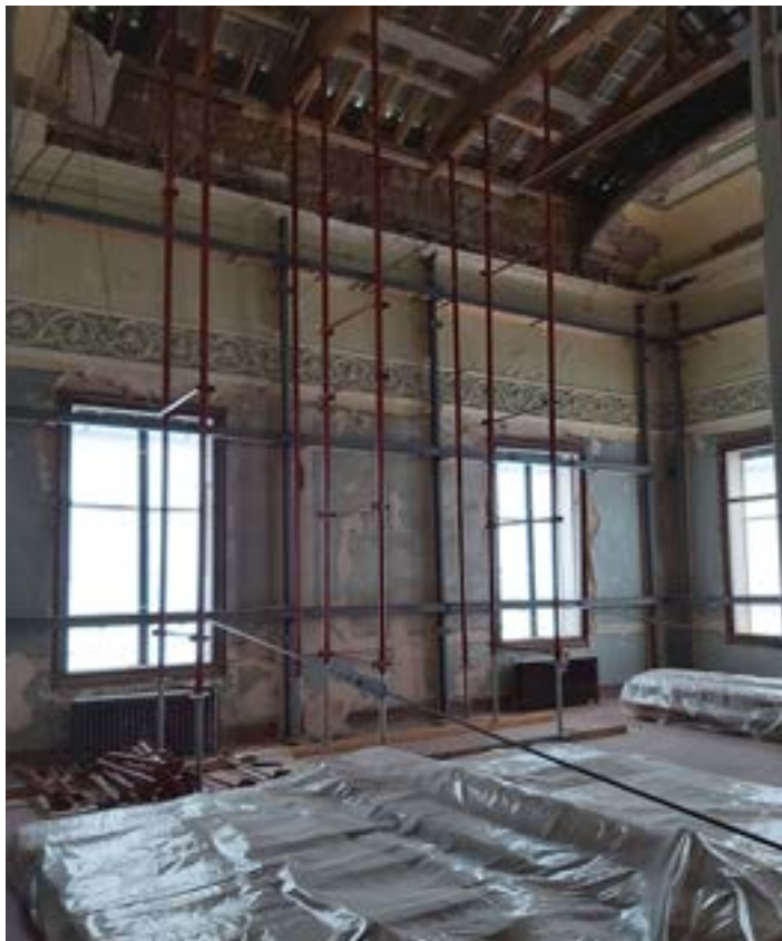
Interior propping and bracing, Y. Dagher
