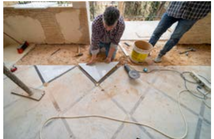
Replacing the broken Carrara tiles, D. Mrad
