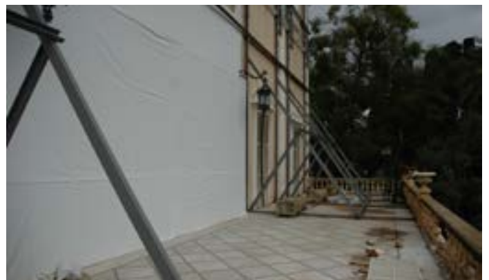
The shoring system standing on the balcony-terrace, Y. Dagher
