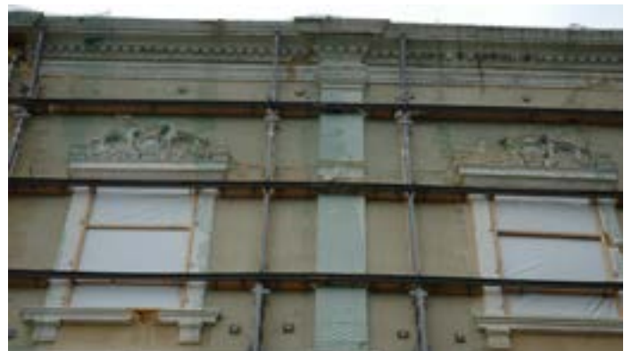
The bracing system on the facade, Y. Dagher
